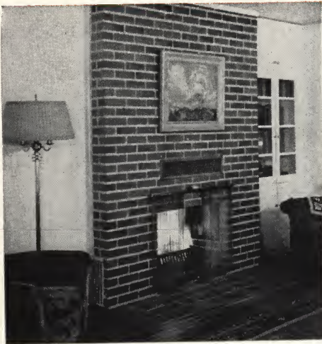
1. Cool Air Intakes At Sides. Warm Air Outlet On Front. (or on side, if desired).
